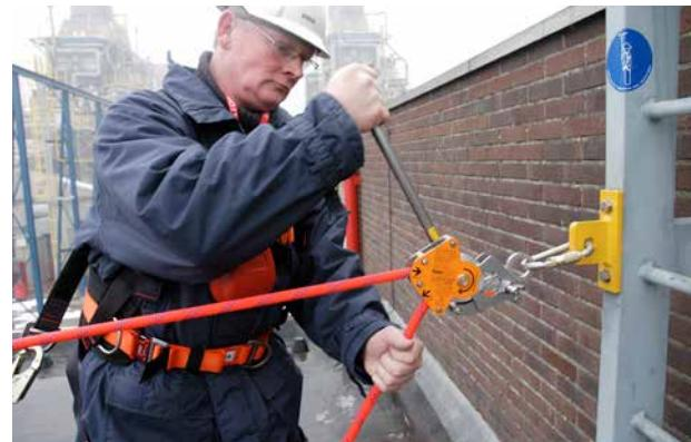
The HONORope-T to be connected with carabiners (min. SWL >20 kN) to the (structural) anchor points. The Rope Vice Tensioner with the tensioning tool provides the right amount of (pre)tension in the HONORope-T system.
