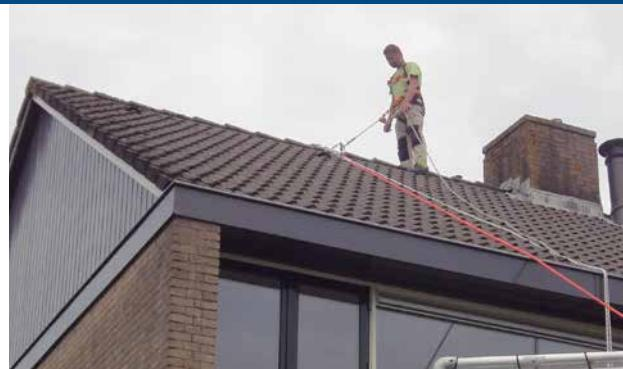
**Anchor.** Central at the (highest available) anchor point for max. 3 Lifelines (users) on the object. Thereafter the Roof-Rope will be tensioned at the front and back side of the object with the Rope Vice Tensioners. Every user connects to a separate Lifeline with his Automatic Rope Grip Device (attached to his safety-harness), which moves along with the user. In case of a fall the Rope Grip Device will block and arrest the user.
