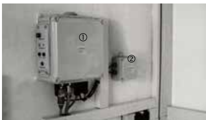
① Control unit - 8.300.01-1 ★ with ② power pack - 8.907.01-1 ★
