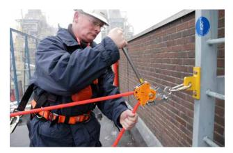
The HONORope-T to be connected with carabiners (min. SWL >20 kN) to the (structural) anchor points. The Rope Vice Tensioner with the tensioning tool provides the right amount of (pre)tension) in the HONORope-T system.
