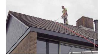
Anchor. Central at the (highest available) anchor point for max. 3 Lifelines (users) on the object. Thereafter the Roof-Rope will be tensioned at the front and back side of the object with the Rope Vice Tensioners. Every user connects to a separate Lifeline with his Automatic Rope Grip Device (attached to his safety-harness), which moves along with the user. In case of a fall the Rope Grip Device will block and arrest the user.
