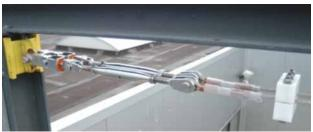
Life Line Tension Indicator for each cable, with Pitchfork, Tensioners & (plastic) Cable Spreader
